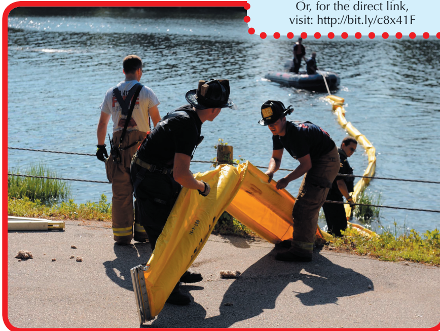
Firefighters work to extend an oil containment boom across the Mystic River June 25 after a tractor trailer struck a guard rail, rupturing its saddle tank, which then fell into the river.
